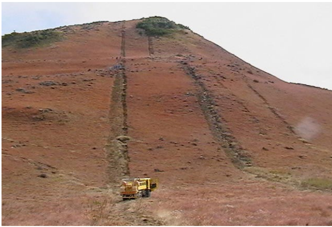
Figure 2: Fire belt constructed parallel to the slope but where two slope aspects meet
